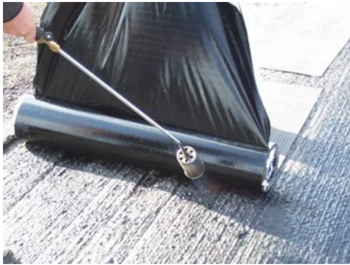
Figure 1 Heating the membrane whilst removing the backing foil
