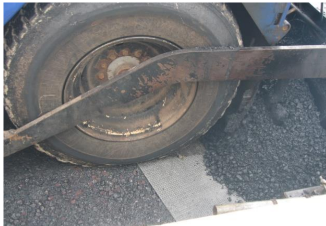
Figure 2 Paving over installed GlasstexPatch Asphalt Interlay
