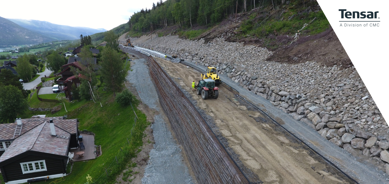
TensorTech GreenSlope reinforced earth slope system delivered a cost-effective alternative for constructing the rockfall protection bund, using locally-sourced fill.
